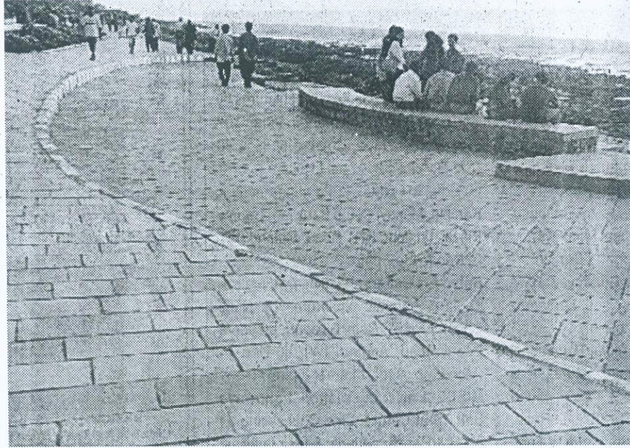
Bandra Bandstand after the redevelopment work
