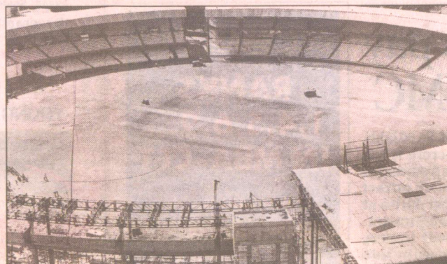
ACTION REPLAY: The Wankhede under construction in 1974 (top) and the completed stadium (above)
