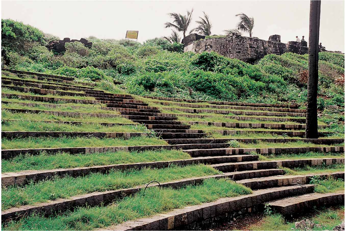
An amphitheatre built on Land's End Hill as part of the redevelopment plan
