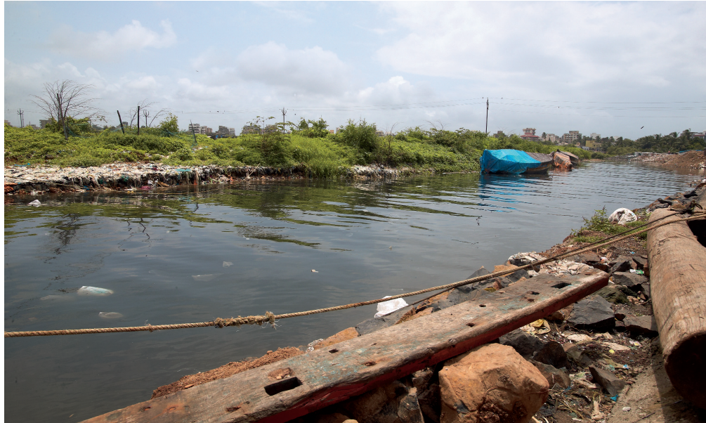
Left: Khar- Danda Creek - Yet another example of neglect and abuse of the waterfronts.
