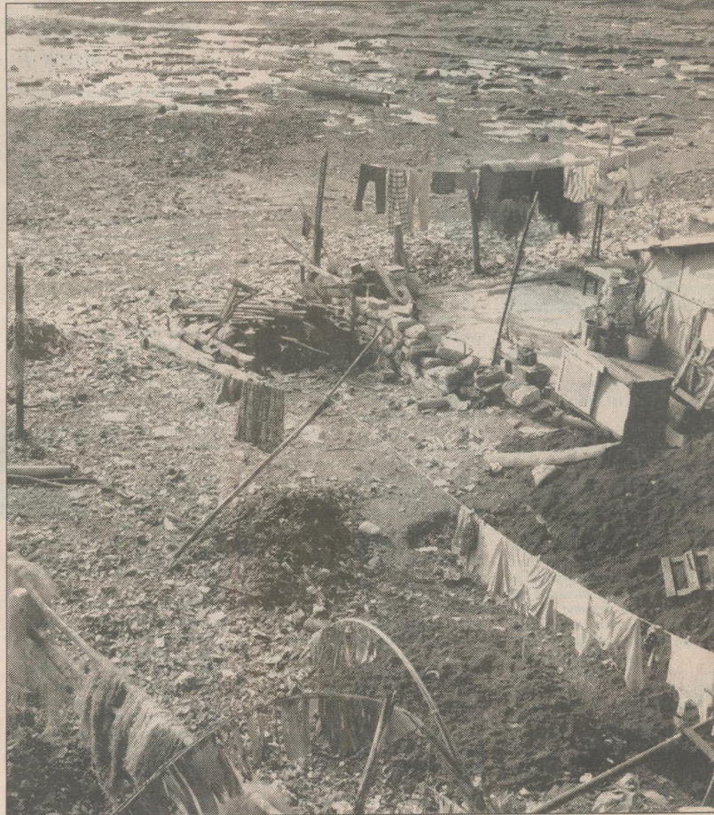
The site for an illegal building, the construction of which was thwarted by alert residents and the authorities
