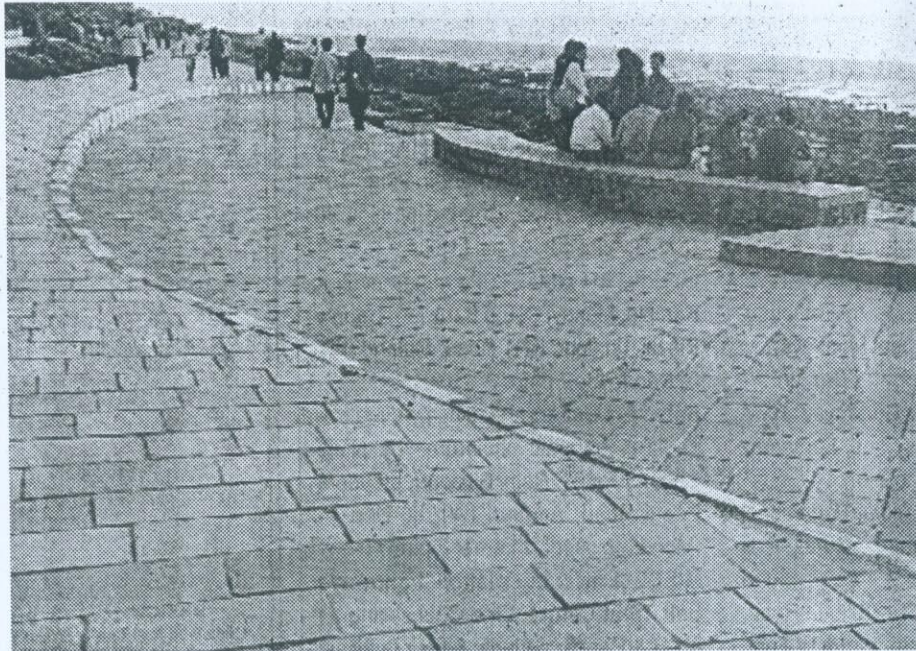
Bandra Bandstand after the redevelopment work
